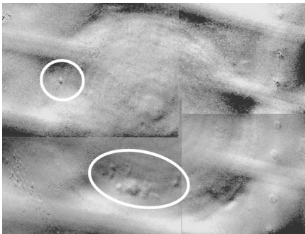
Photo8 Another application of thermal shearography is the inspection of scarf-joint repairs to solid composite laminate aircraft structure. Here porosity is detected. Bonded stringers on the far side surface are seen as the diagonal linear
